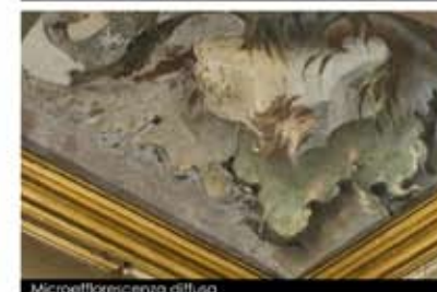
Microefflorescenza diffusa
